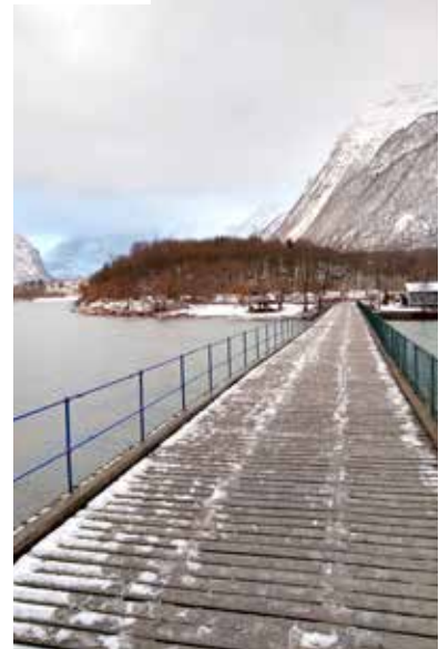
Footbridge over Rauma River
